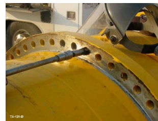
Cleaning paint and rust prior to torquing
