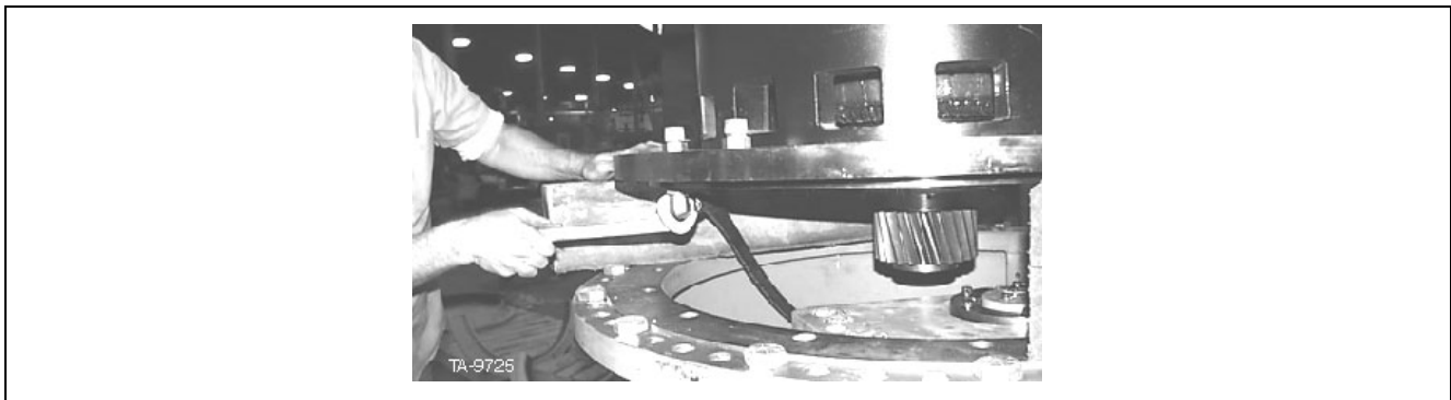
Figure 28. Disconnection of oil return hose
